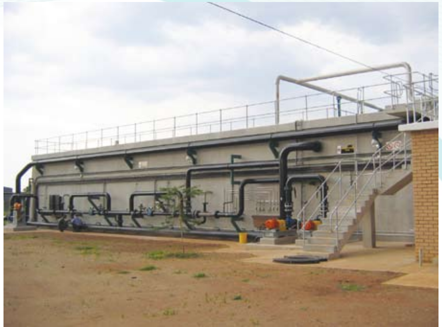
One of the anaerobic digesters used by Talbot & Talbot
